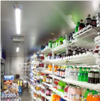
Walk-in cooler lighting
